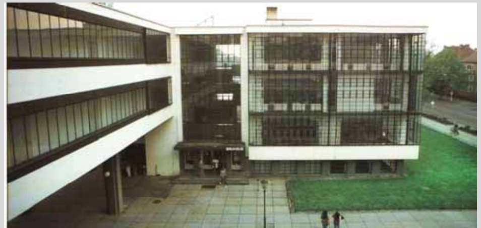
Bauhaus Buildings in Dessau (1925-26) by Walter Gropius
