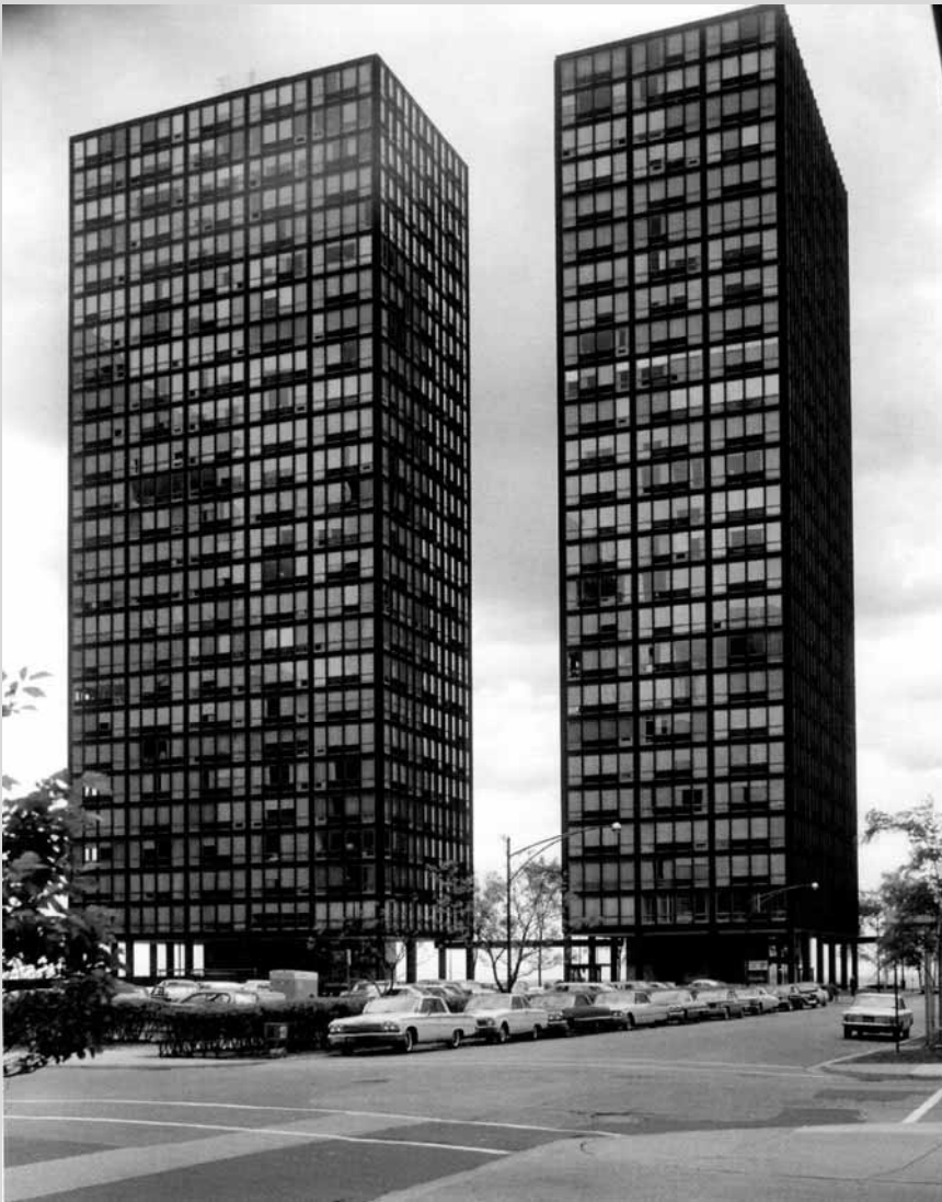
Lake Shore Drive Apartment, Chicago, Illinois (1948-51)
